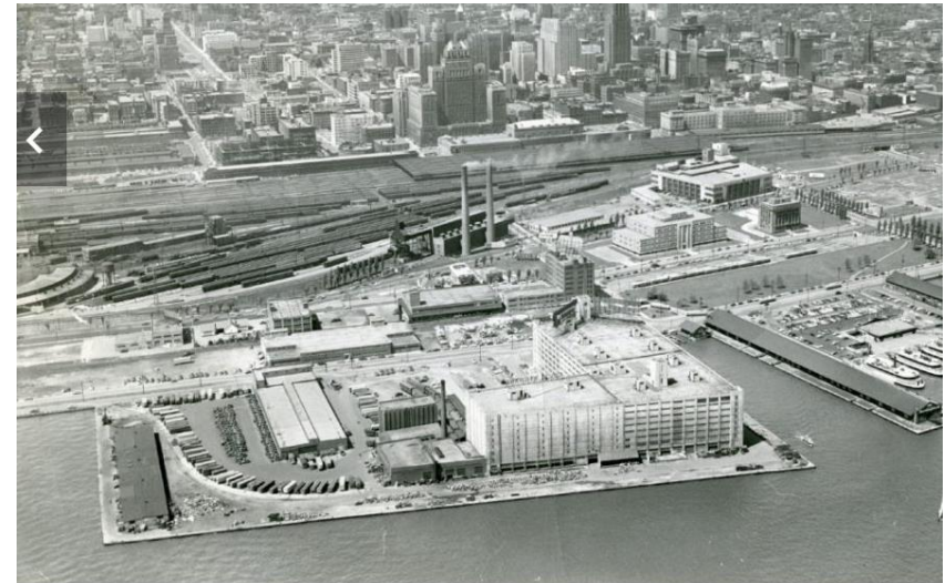
Before the Gardiner Expressway, the lakefront area of Toronto had a very different look in 1954. The expressway construction began in sections until 1964. (TORONTO STAR FILE PHOTO)
